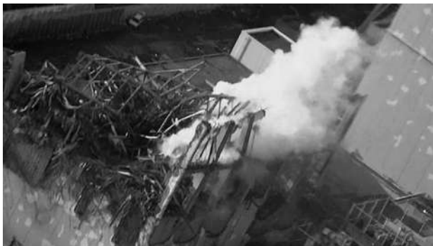
Рис. 30. Figure: Collapsed reactor building of Fukushima
