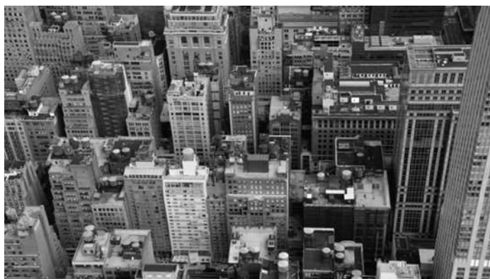
Рис. 20. Figure: Water tanks on buildings in New York, as seen from the Empire State Building
