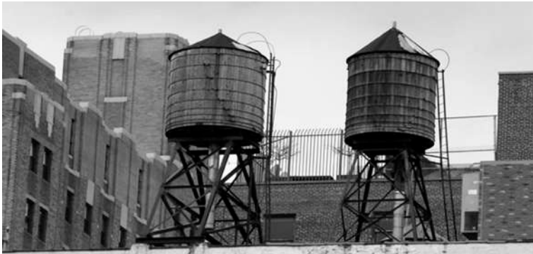
Рис. 21. Figure: Typical rooftop water tanks in New York City
