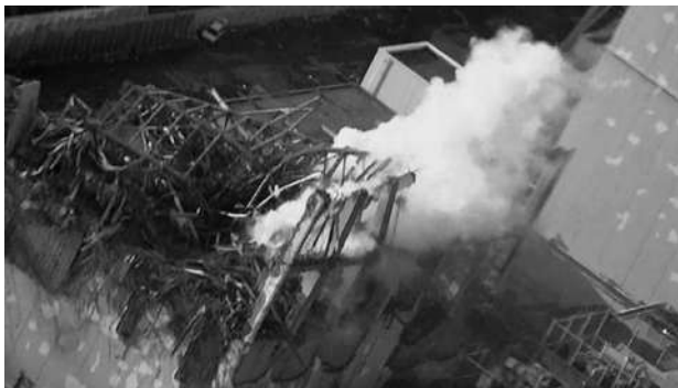
Рис. 30. Figure: Collapsed reactor building of Fukushima
